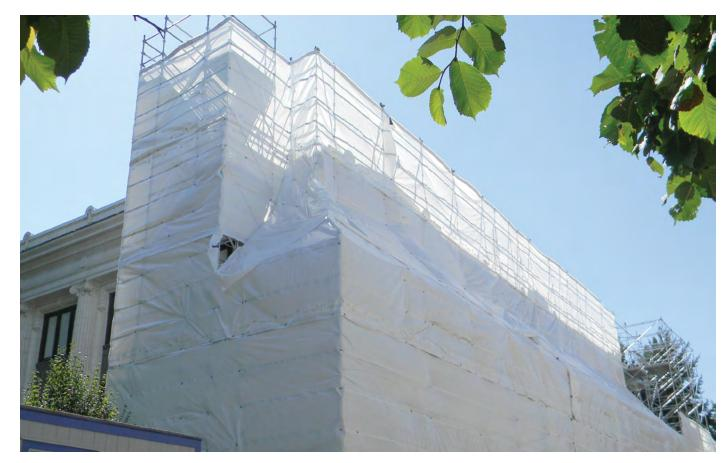
Supreme Court Building scaffolding on the north facade is draped with dust covering during rehabilitation work.
